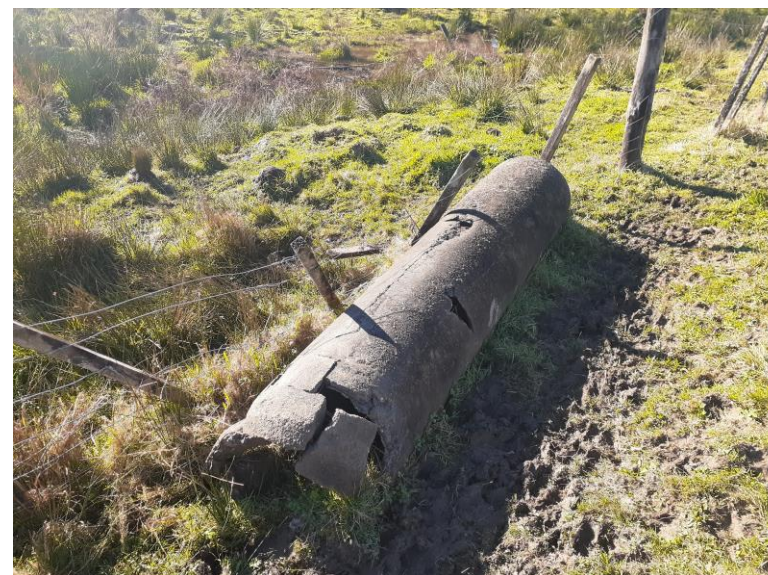
Old damaged culvert Southeast of existing culvert
